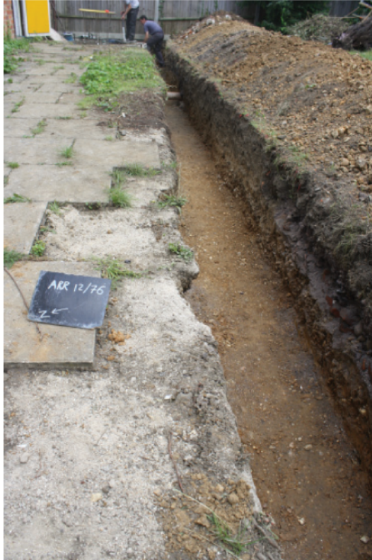
Plate 1. General view of footing trench, looking north east.
