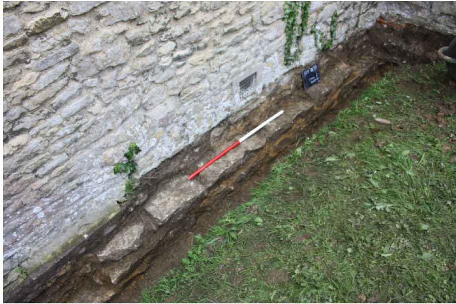
Plate 3. Faced blocking in foundation, looking south east, Scale: 1m.
