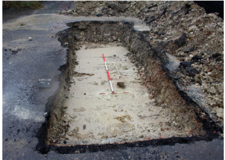
Plate 2. Trench 2, looking north, Scales: 2m and 0.5m.
