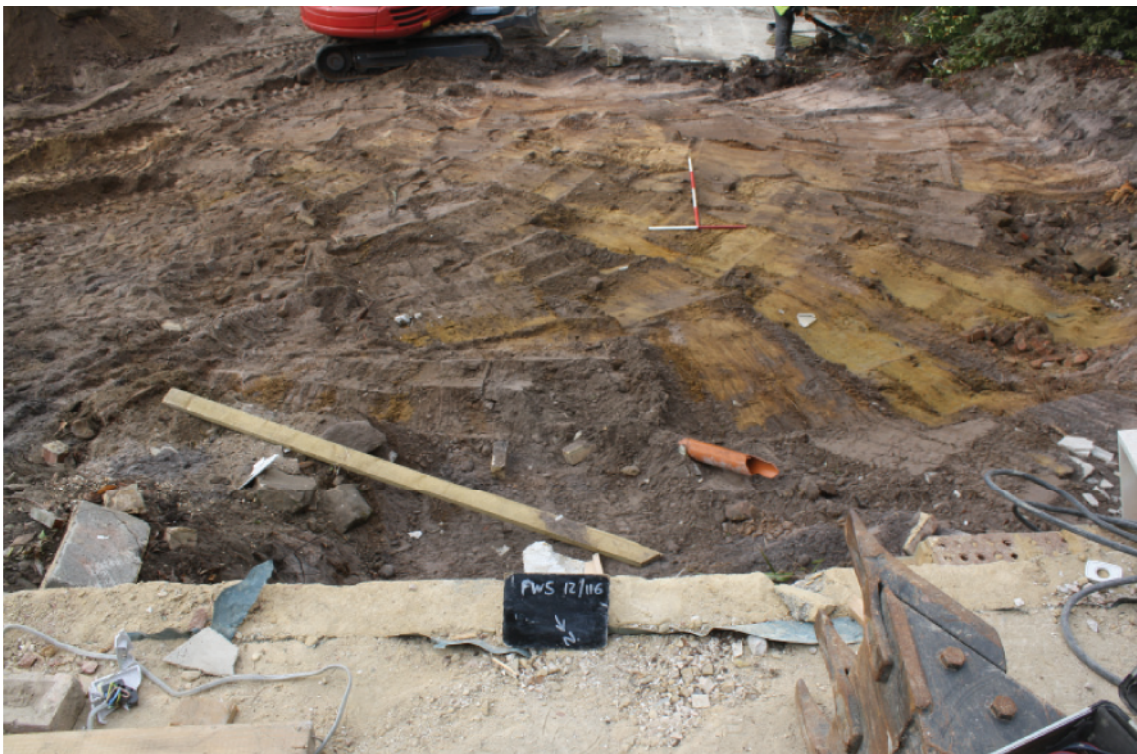
Plate 2. House strip, looking southwest, Scales: 2m and 1m.
