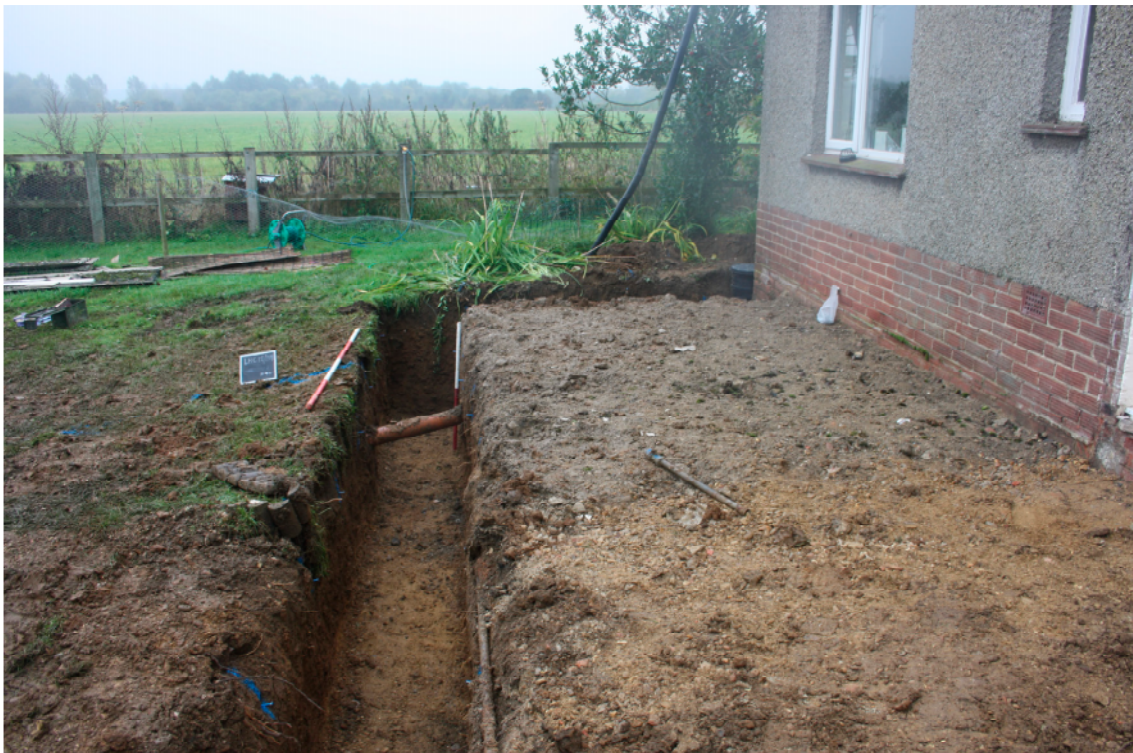
Plate 1. Footing trench, looking east.
