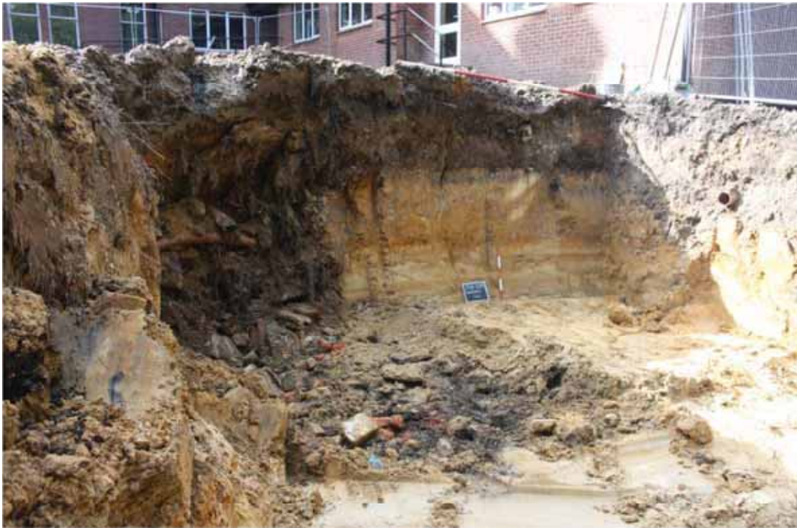
Plate 1. Plant room footings excavation, looking west, Scales: 2m and 0.5m.
