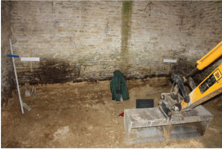
Plate 1. Reduction of floor within barn
