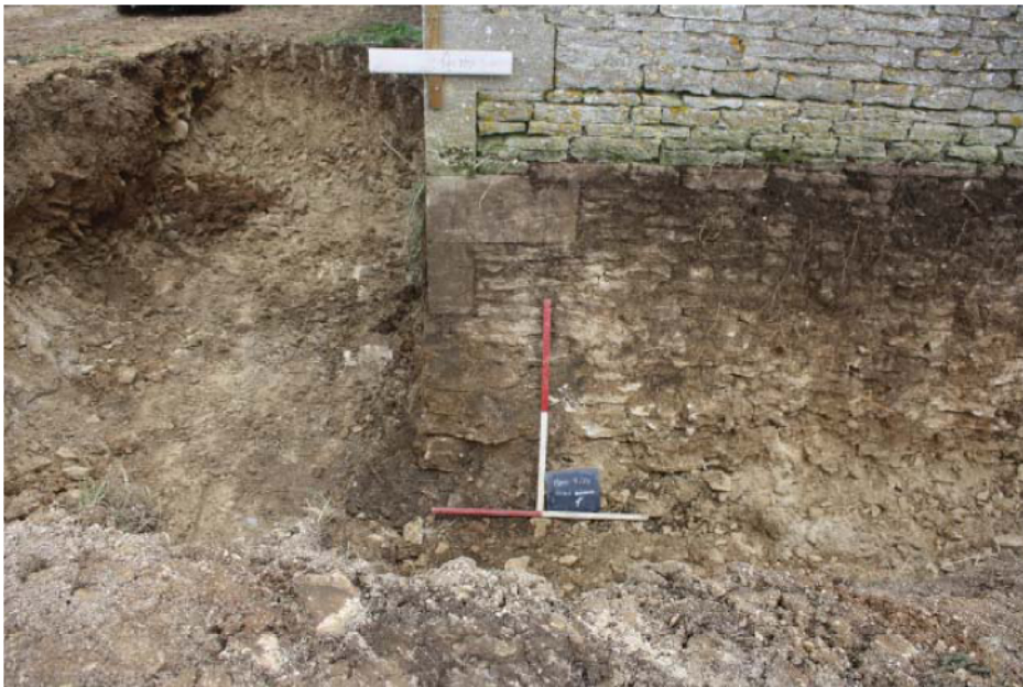
Plate 2. Exterior of barn showing exposed footings. looking west. Scales: 1m
