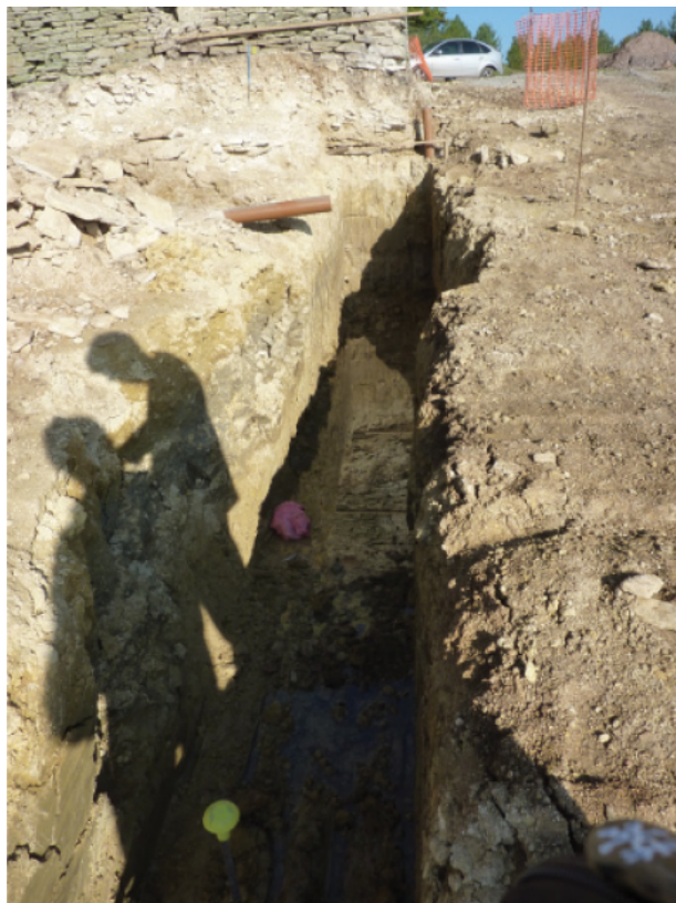
Plate 3. Footing trench for external wall, looking west
