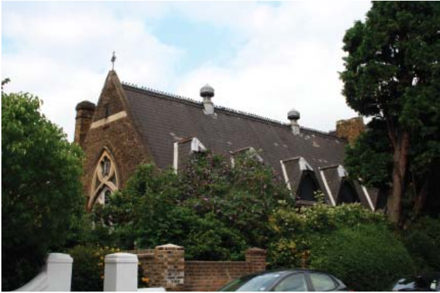
Plate 1. Exterior, elevation of southwest corner of room 11, looking northeast.
