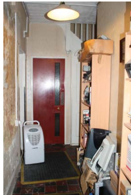
Plate 16. Interior, ground floor, room 3, looking east.
