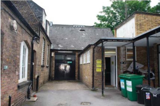
Plate 9. Exterior, east elevation, rooms 23, 10, 15 and 22, looking west.
