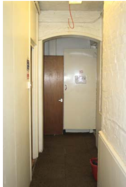
Plate 14. Interior, ground floor, room 1, looking south.
