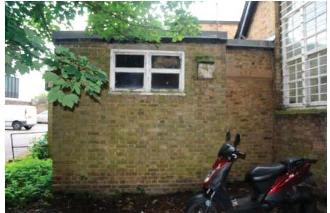
Plate 6. Exterior, west-facing elevation of room 18, looking east.
