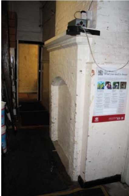
Plate 25. Interior, ground floor, room 15, detail of bricked-up fireplace, looking northeast.
