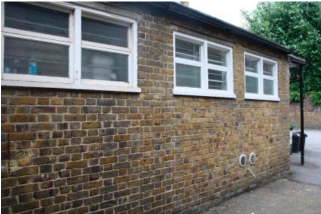
Plate 5. Exterior, south-facing elevation of room 22, looking northeast.
