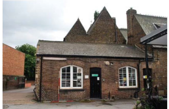
Plate 10. Exterior, north-facing elevation of room 7, looking south, scales 2.0m.
