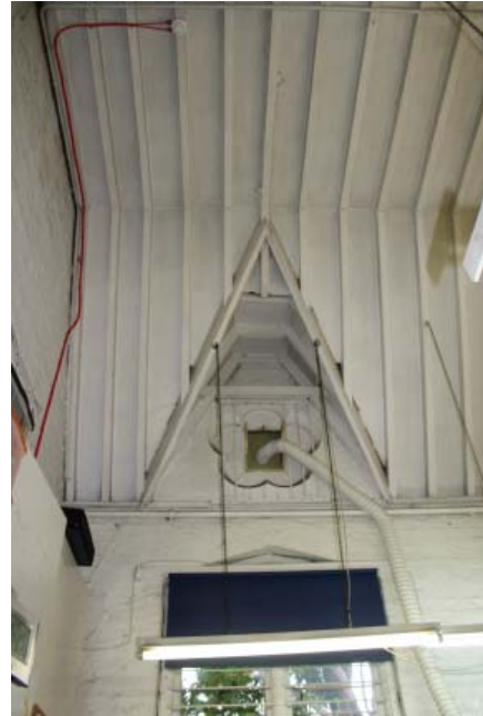
Plate 22. Interior, ground floor, room 9, detail of ceiling, looking south.
