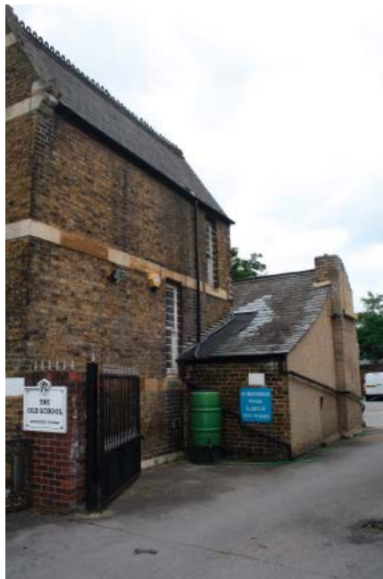
Plate 7. Exterior, east elevation, rooms 4 and 7, looking northwest.
