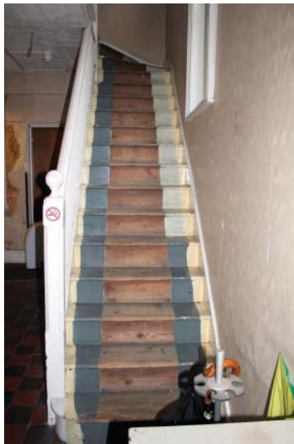
Plate 19. Interior, staircase to first floor, room 4, looking north.
