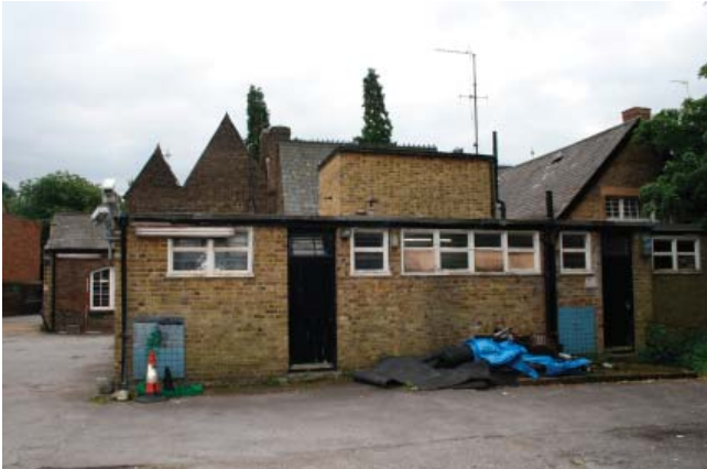
Plate 13. Exterior, north-facing elevation of rooms 20, 19 and 18 looking south.
