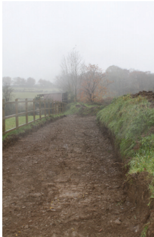
Plate 2. Access Track looking south west.
