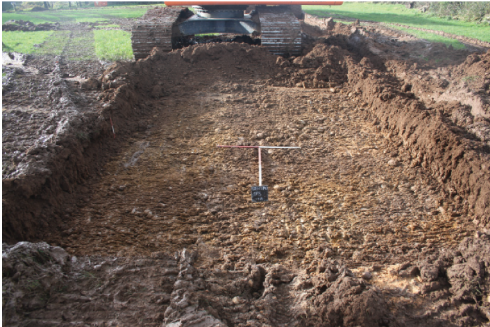
Plate 1. TP 3 looking west, Scales: 1m.
