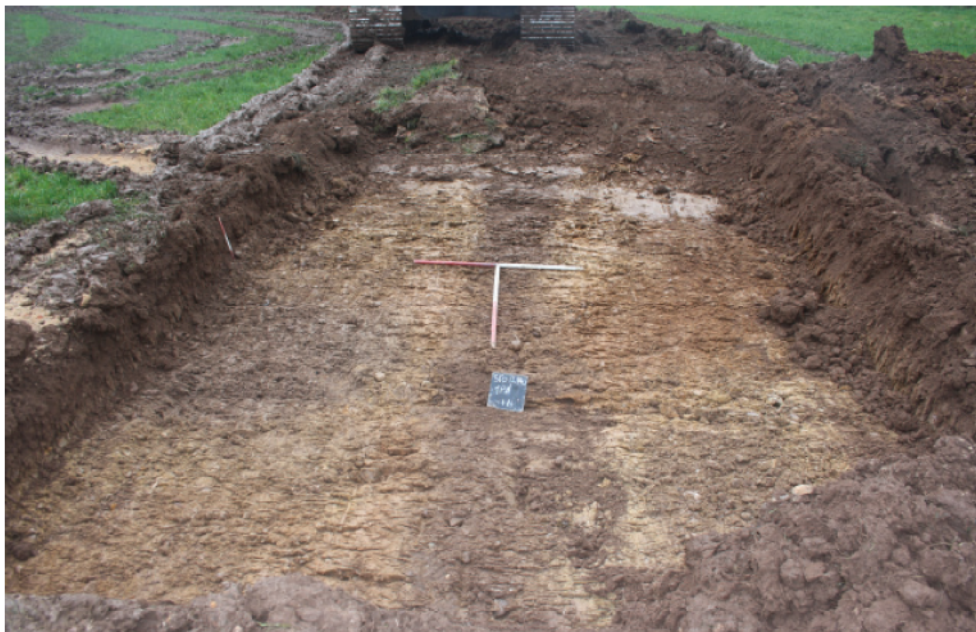
Plate 2. TP 4 looking west, Scales: 1m.
