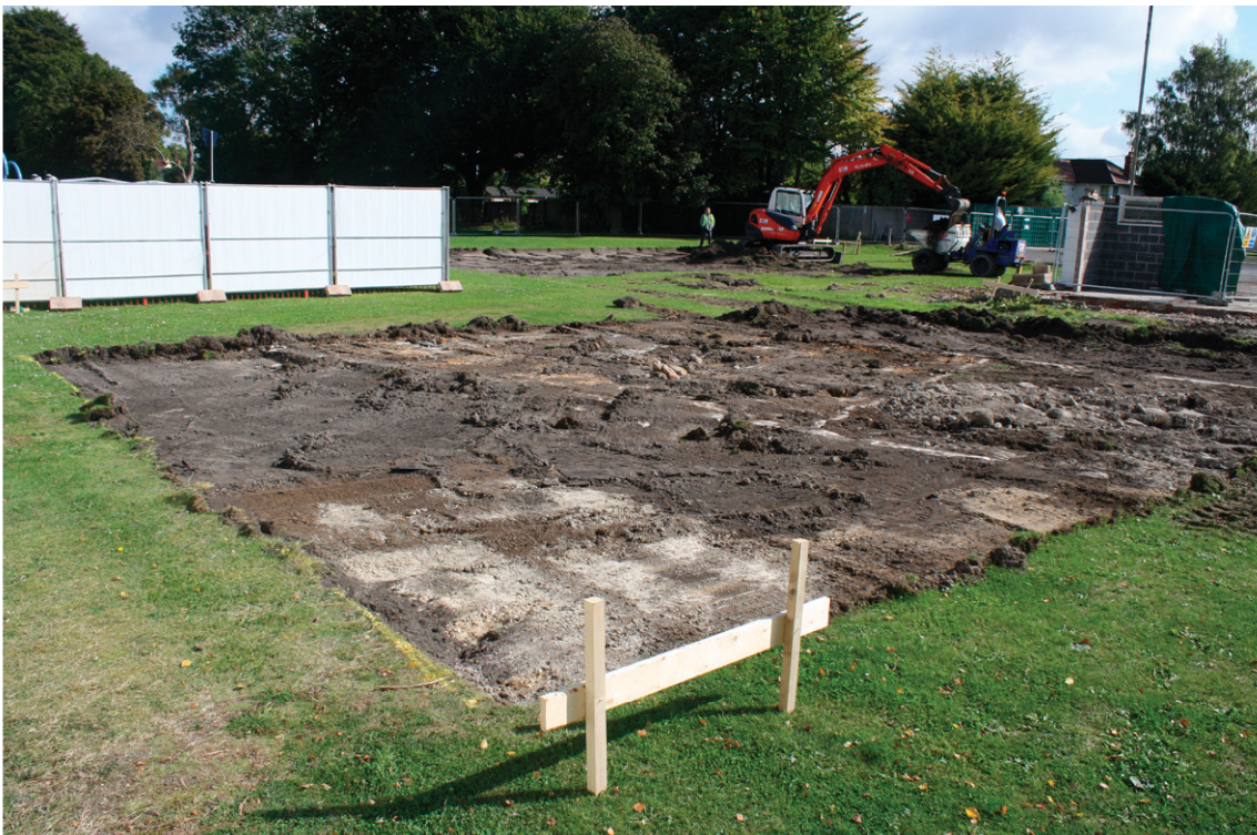
Plate 1. Turf stripping across the site, looking east.
