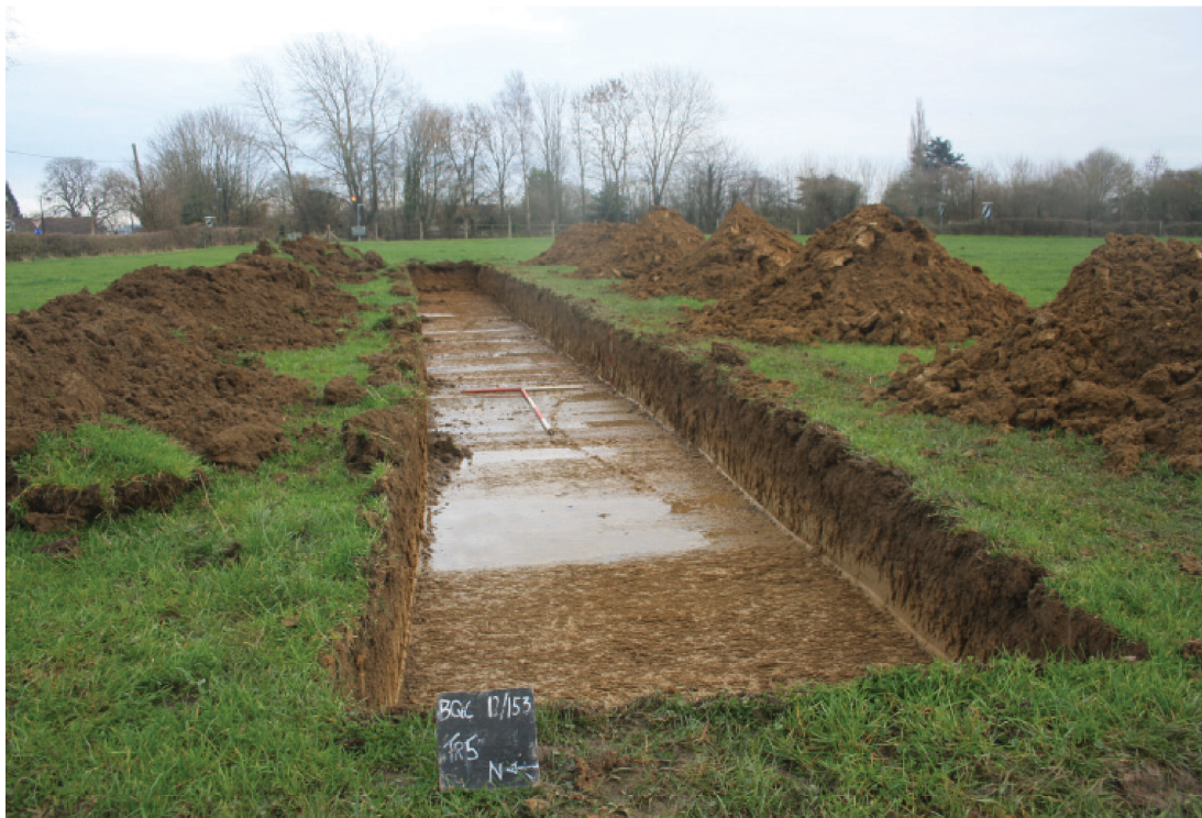
Plate 2. Trench 5 looking east. Scales: 2m, 1m and 0.5m
