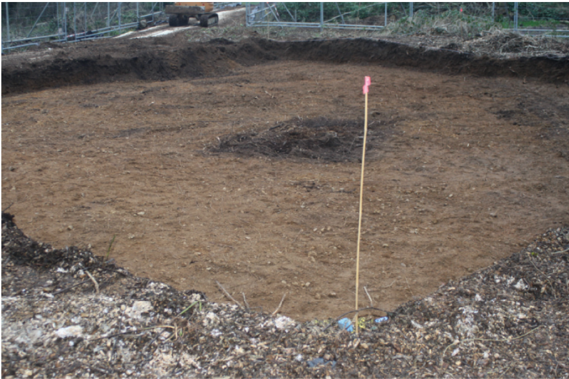
Plate 1. General view of area stripped for mast location, looking south east.
