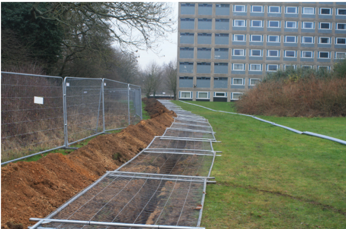
Plate 2. General route of cable trench, looking north east towards Sibley Hall.
