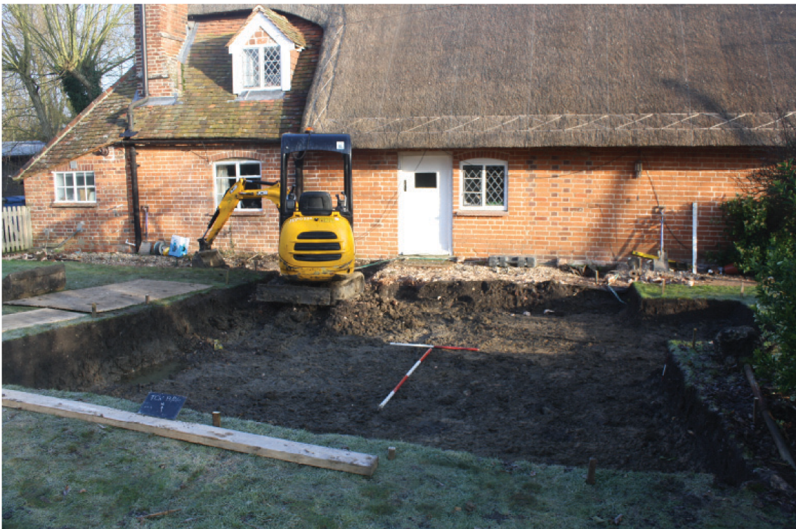
Plate 1. Stripped area, looking north, Scales: 2m and 1m.
