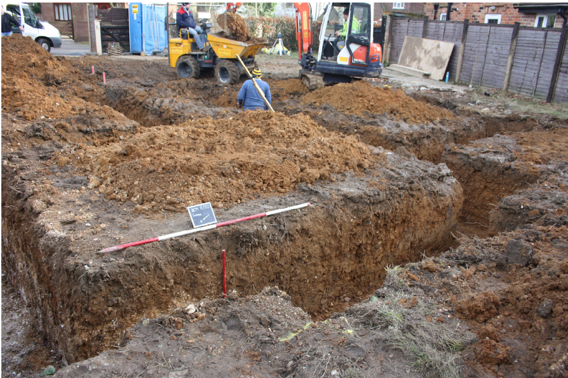
Plate 1. New footing trenches, looking south east, Scales: 2m and 1m.
