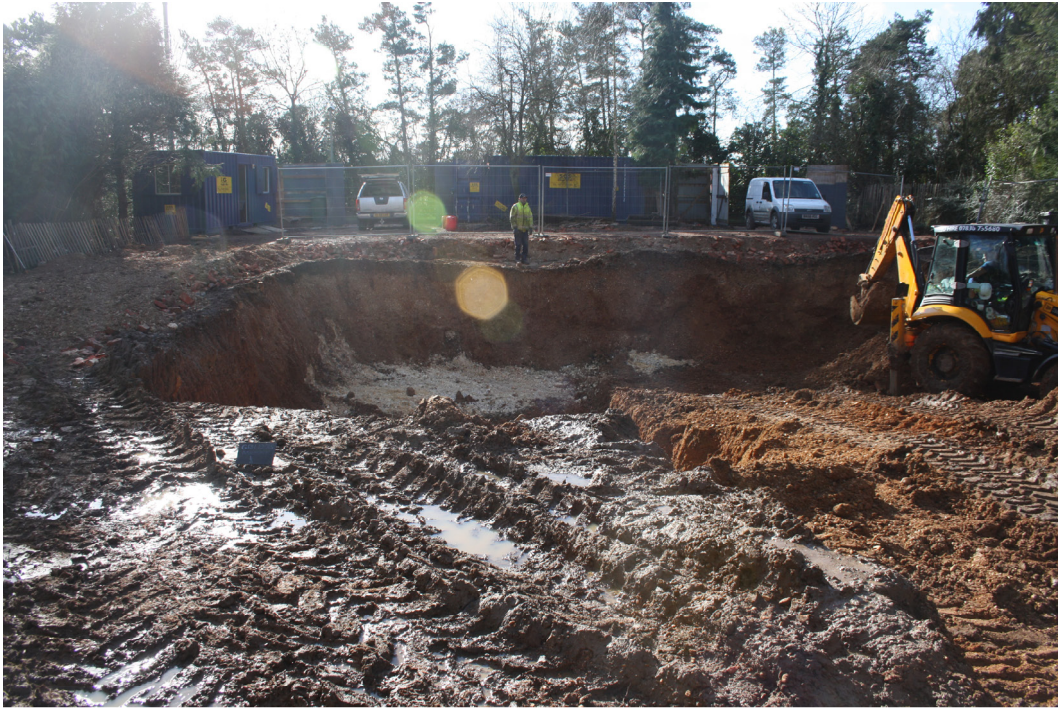
Plate 3. General view of site looking north.
