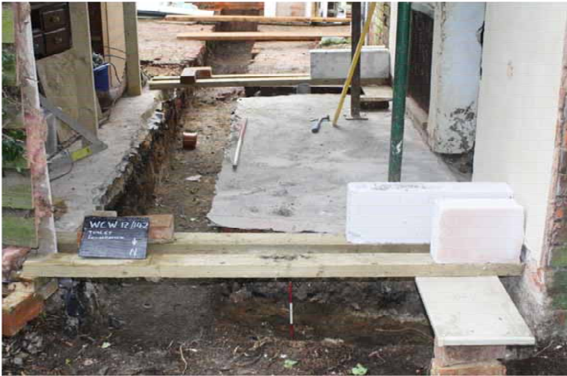
Plate 1. New foundation trench, looking south, Scales: 1m and 0.3m.
