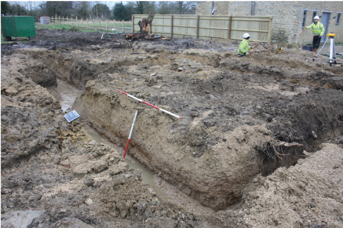
Plate 1. Plot 2 footing, looking north east, Scales: 2m and 1m.
