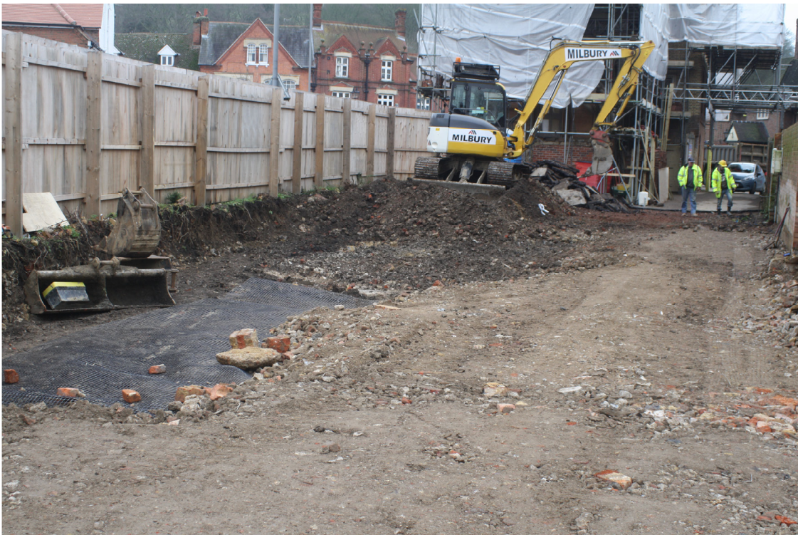
Plate 1. Laying of piling mat, looking east.
