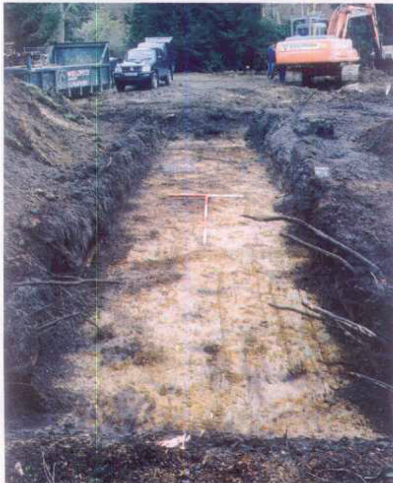
Plate 2. Trench 2 looking north, scales 2m, 1m.
