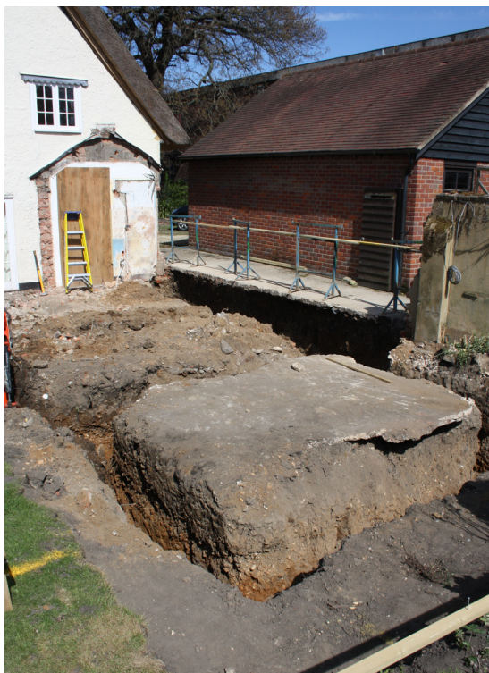
Plate 2. Rear extension and conservatory footings, looking north.
