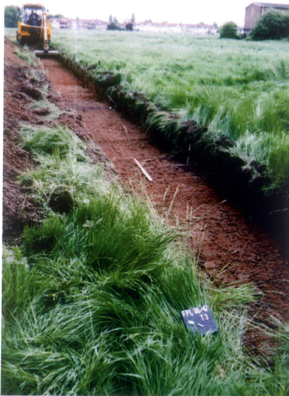
Plate 1. Trench 3 looking north east, vertical scale 0.3m, horizontal scale 1m.
