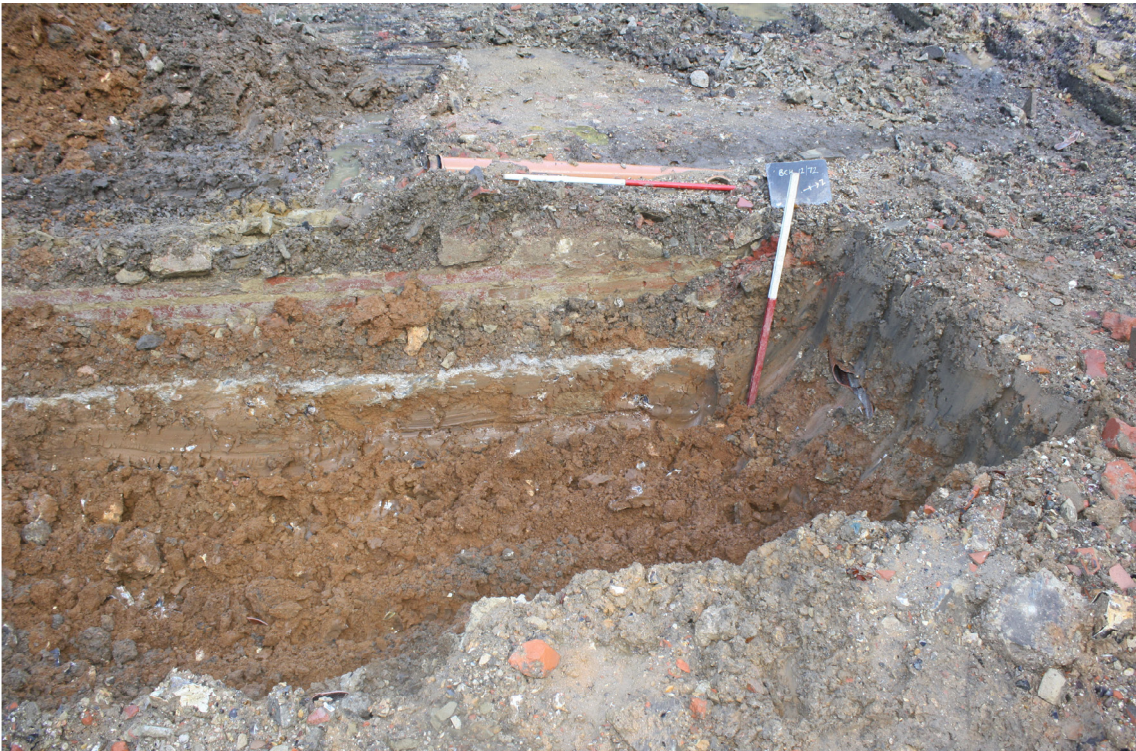
Plate 2. Excavation by side of existing foundation before removal, looking north west, Scales: 1m.
