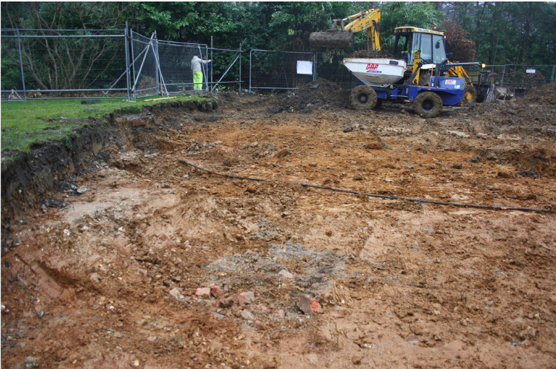
Plate 1. Northern edge of area of ground reduction, looking east.
