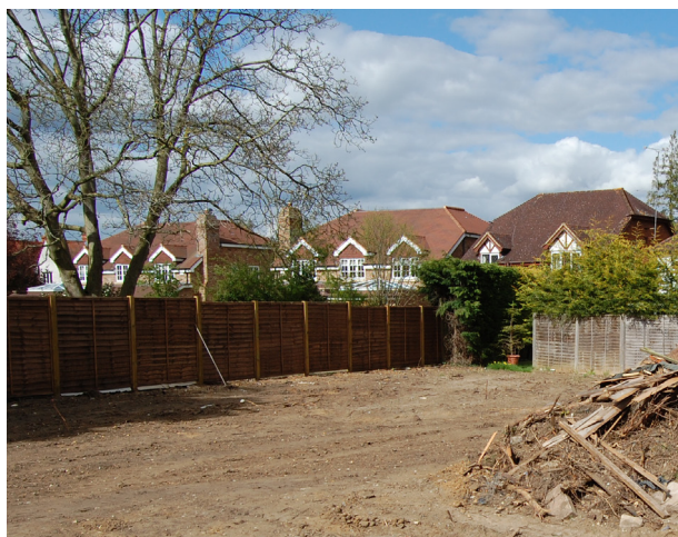
Plate 1. General view of site looking north-east.
