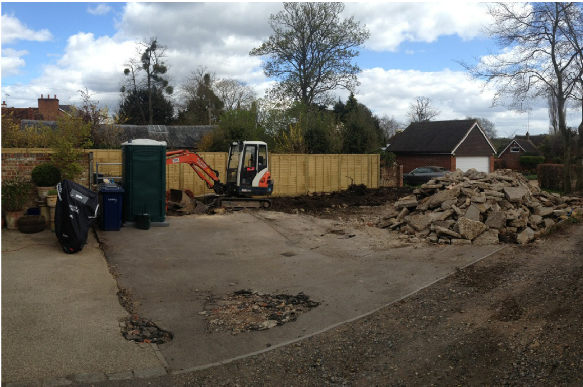
Plate 1. Site view, during concrete slab removal. looking south east
