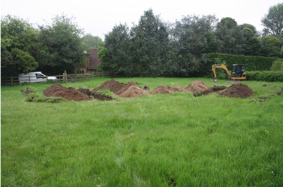
Plate 1. Location of trenches, looking south.
