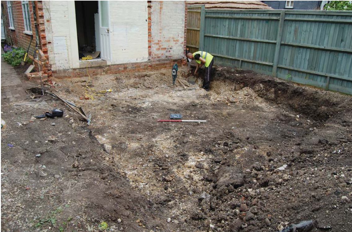
Plate 2. Reduced strip at rear of cottage, looking north east, Scale; 1m.
