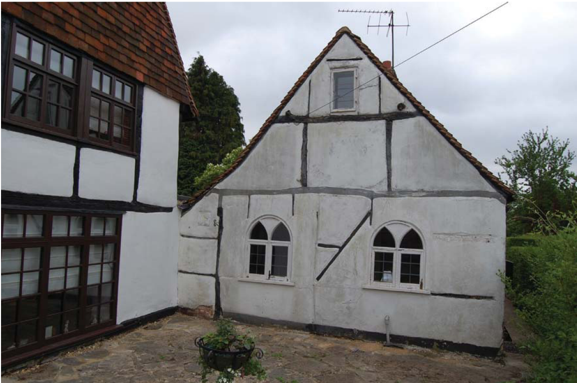
Plate 1. Gable end elevation (front) of the Listed Building, looking south.
