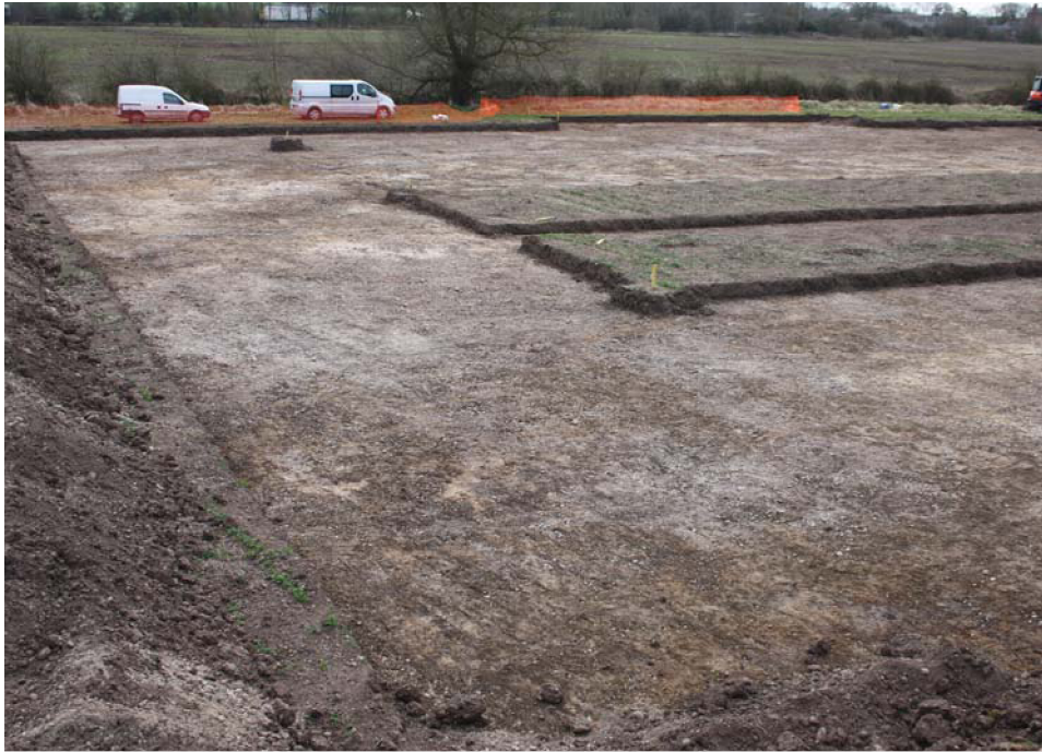
Plate 1. Stripped area, looking north west.
