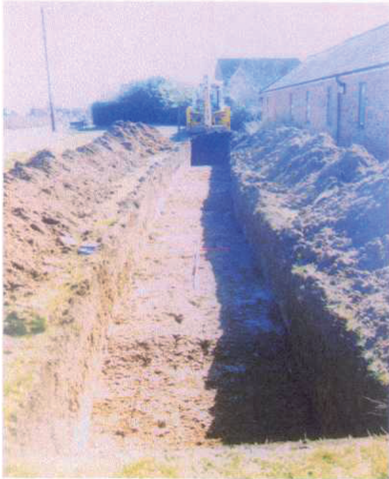
Plate 1. Trench 1, Looking east, scales 2m, 1m.
