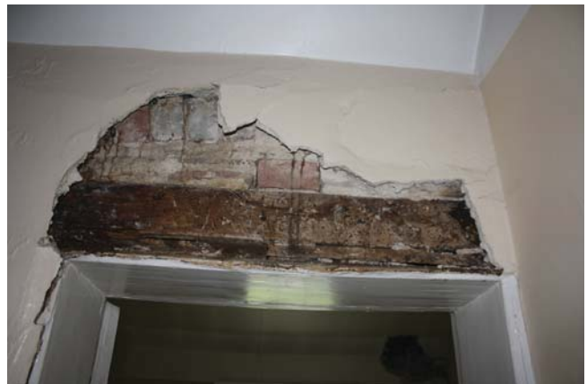
Plate 16. Room 26, oak lintel above doorway to room 21, looking west.
