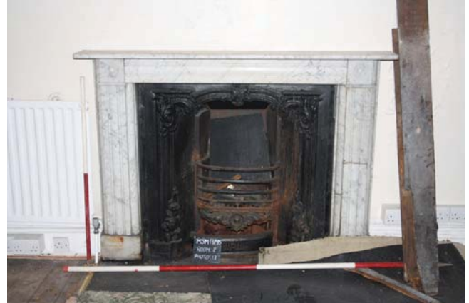
Plate 6. Room 2, detail of fireplace, looking east, Scales: 2m and 1m.
