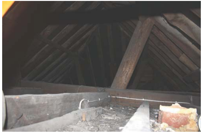
Plate 20. Roof above room 29, looking east.
