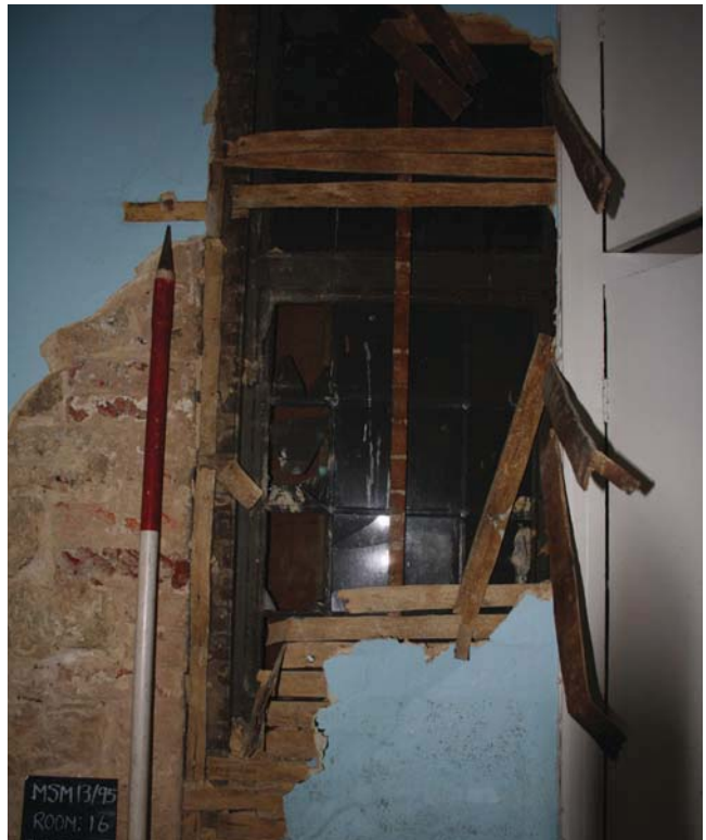
Plate 12. Room 16, view of blocked window, looking west, Scale: 2m.
