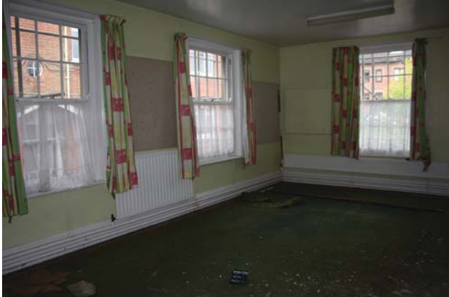
Plate 13. Room 1, view to windows, looking south east, Scales: 2m and 1m.
