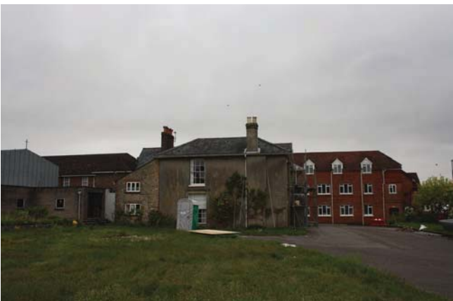
Plate 3. Exterior, side elevation, looking east.
