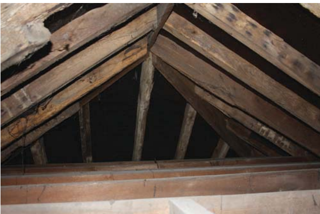
Plate 19. Roof above room 19, looking north.
