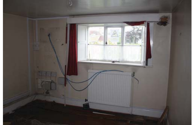
Plate 10. Room 5, view to window, looking south west, Scales: 2m and 1m.
