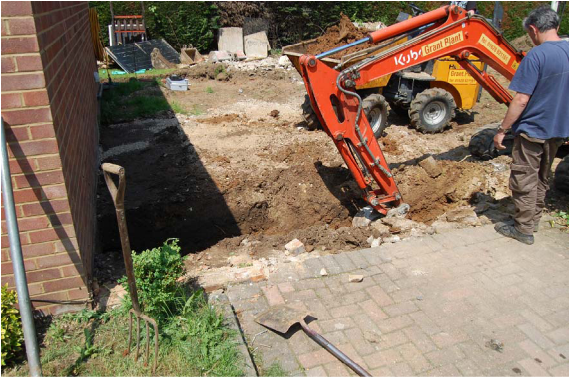
Plate 1. Front of garage (eastern) footing under excavation.
