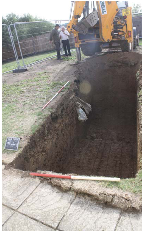
Plate 1. Trench 1 looking south east, Scales 2m and 1m
