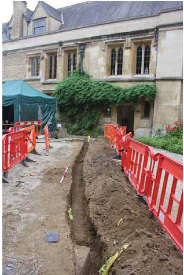
Plate 2. Along the trench, looking north west, Scales: 2m and 0.3m.
