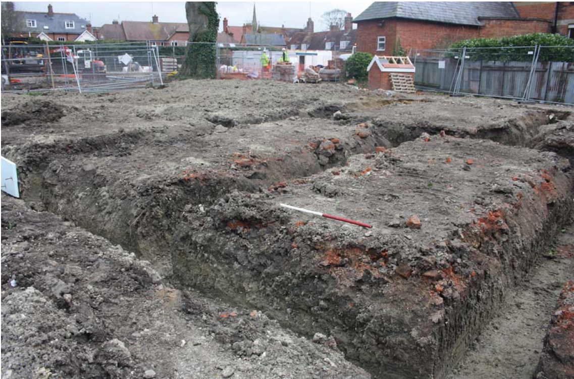
Plate 2. Plot 9 exposed sections, looking north, Scales: 1m.
