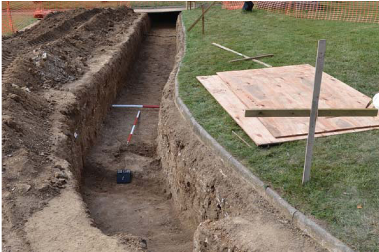
Plate 1. Sewerage trench, looking northwest, Scales: 2m and 1m.
