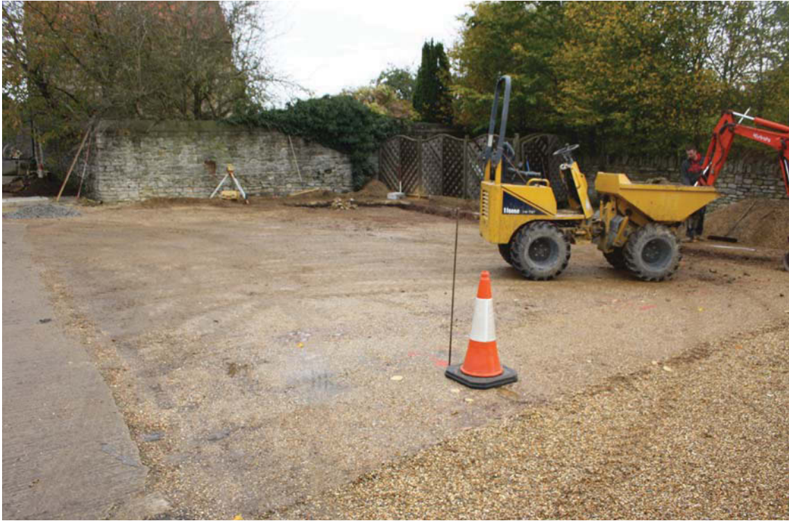
Plate 1. Area of new footing, looking north.
