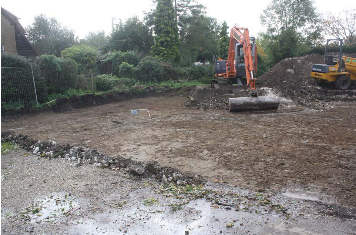
Plate 1. Stripping progress, looking south east, Scales: 2m, 1m and 0.5m.
