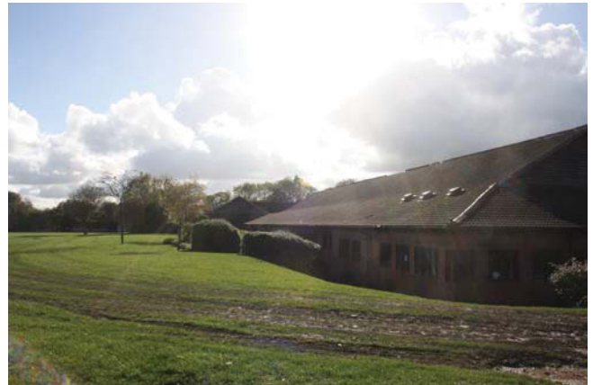
Plate 2. Terracing of school into interior of earthwork.
