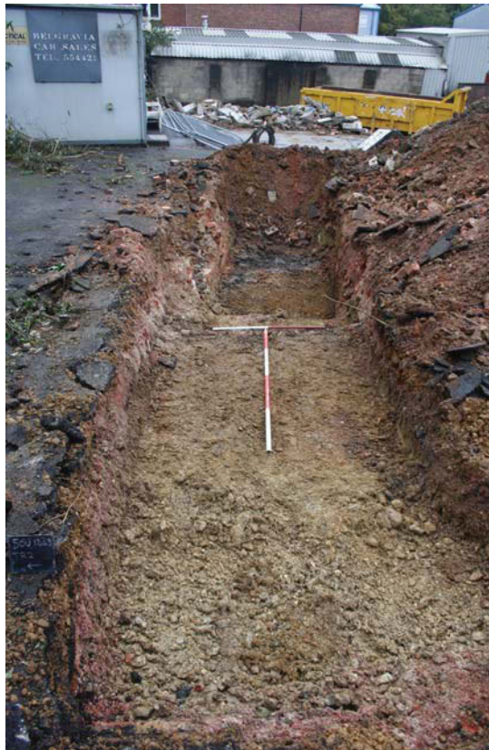
Plate 2. Trench 2, looking south east, Scales: 2m and 1m.
