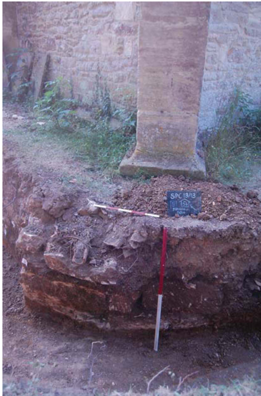
Plate 3. Tower buttress foundation (56) looking south east, Scales: 1m and 0.5m.
