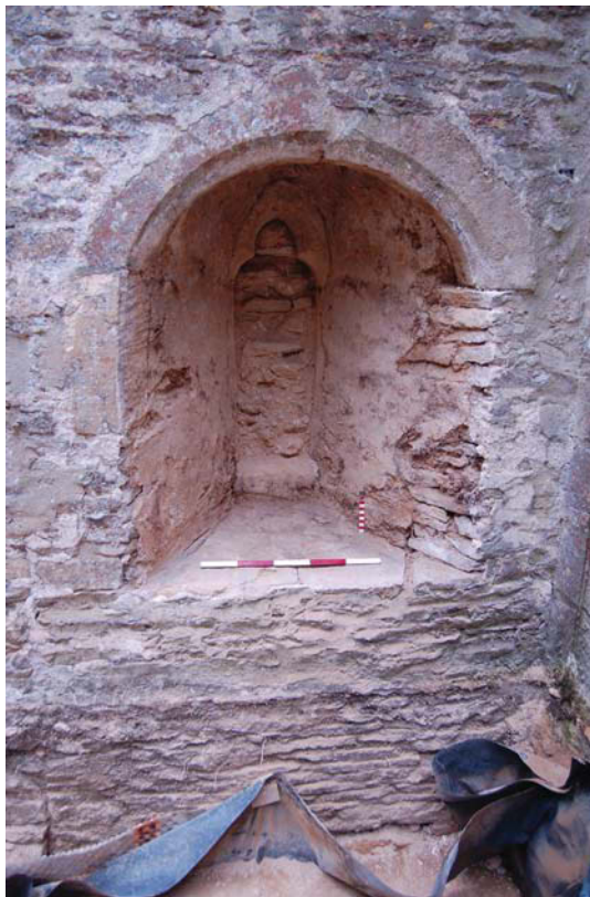
Plate 4. Exposed window, north transept wall, west face, Scales: 0.5m and 0.1m.
