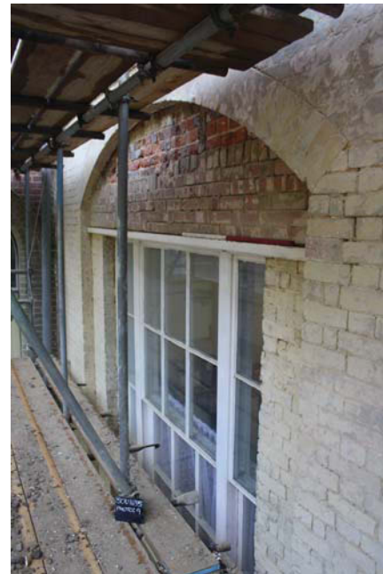
Plate 12. South wing above window, looking south, Scale: 1m.
