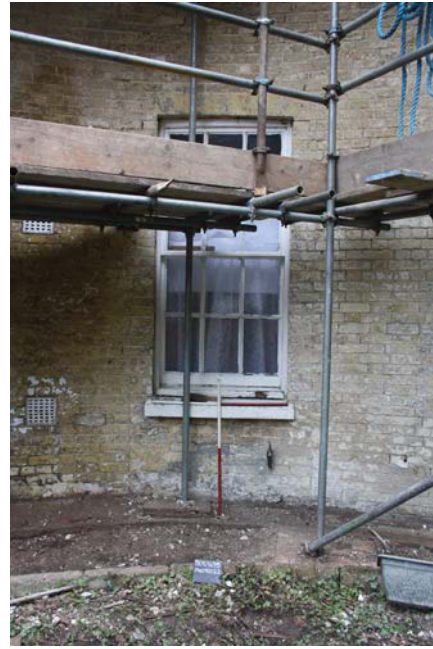
Plate 4. Brickwork under window, N wing, looking west, Scales: 1m.
