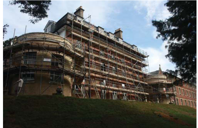
Plate 2. Rear of building, looking east.
