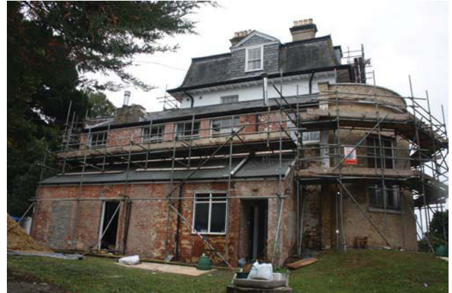
Plate 10. General view lean to, looking north east.
