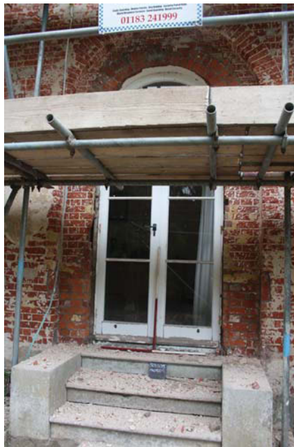
Plate 3. Brickwork around door, looking north east, Scales: 1m.
