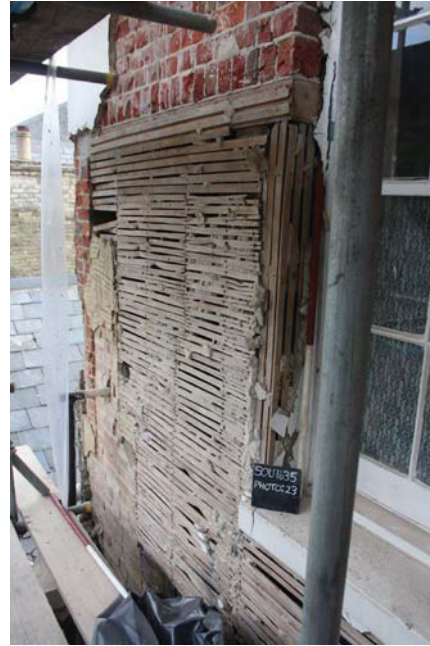
Plate 8. Laths top, South wing, South side, looking south, Scales: 1m.
