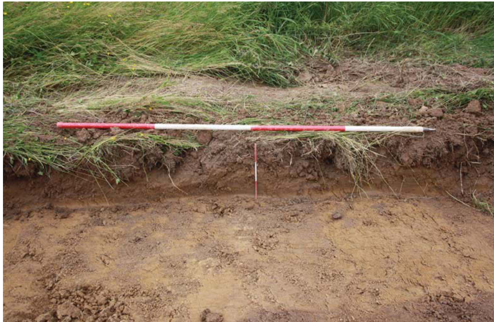
Plate 4. Haul road, section, looking west, Scales 2m and 0.3m.
