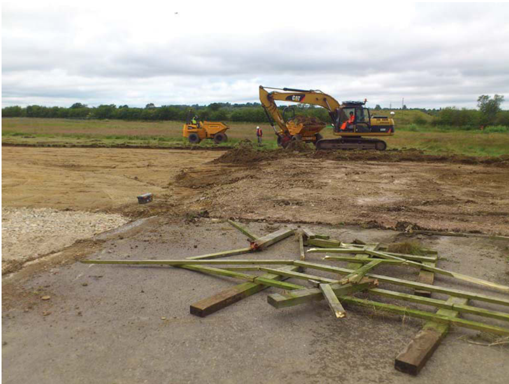
Plate 2. Edge of old compound area, looking west.
