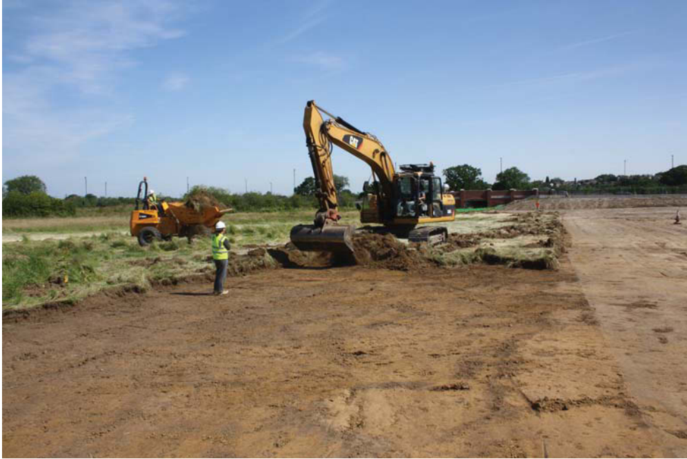
Plate 1. Site strip in progress, looking north.
