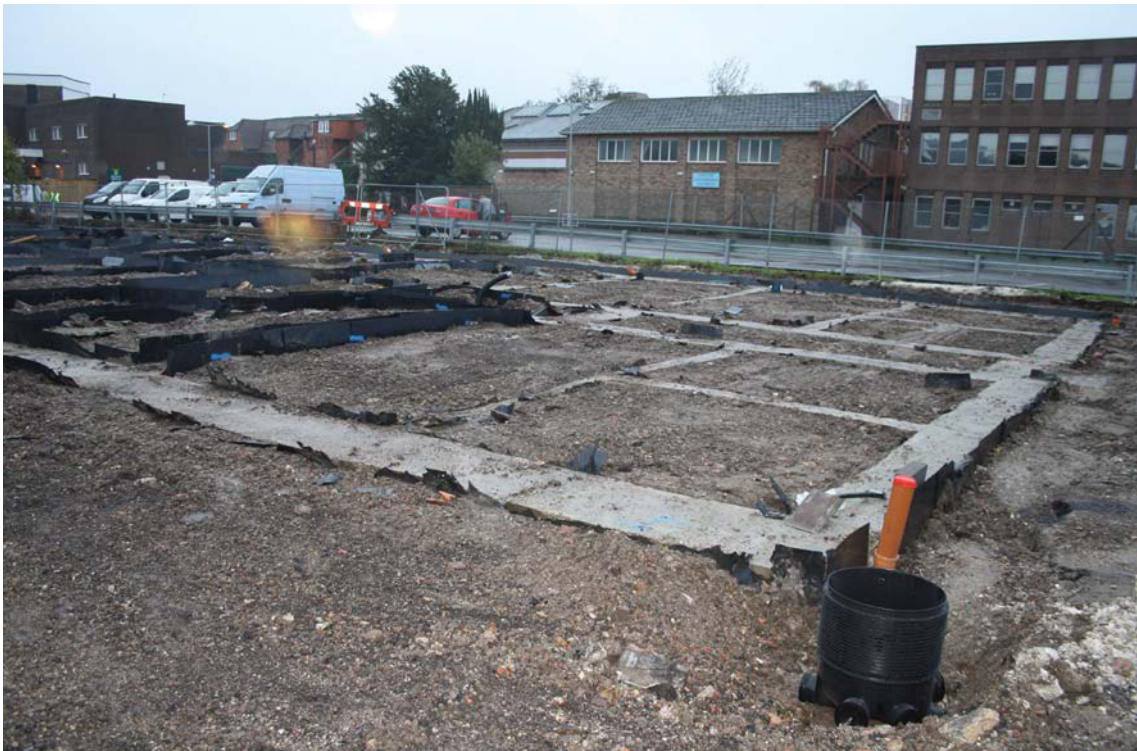
Plate 2. Concreted western aspect of foundation, looking south east.
