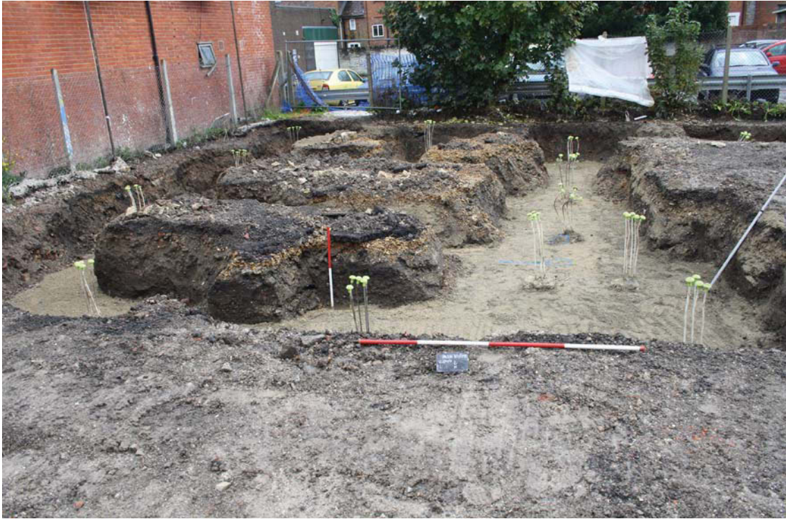
Plate 1. Eastern foundation trenches, looking south, Scales: 2m and 1m.
