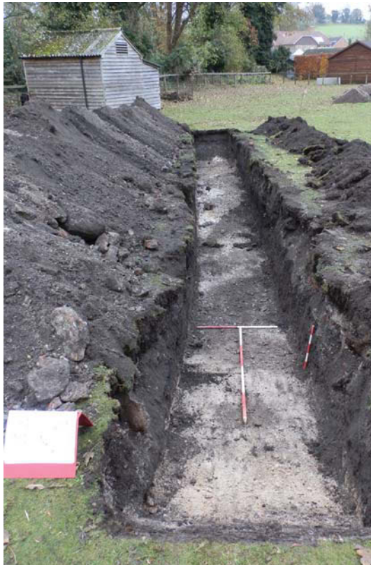
Plate 1. Trench 1, looking north east, Scales: 2m, 1m and 0.5m.
