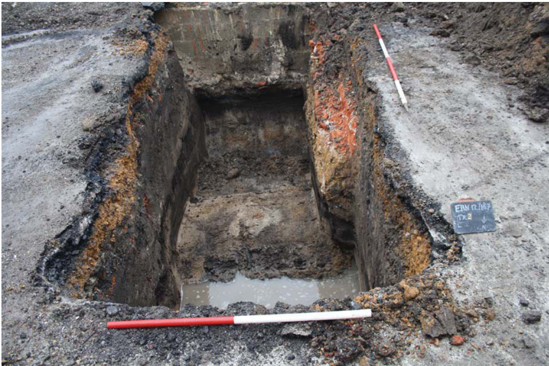
Plate 2. Trench 2, looking south, Scales: 2m and 1m.
