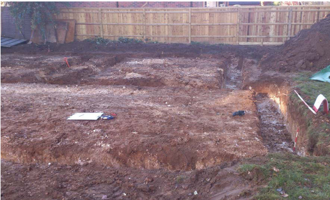
Plate 2. View of footing trenches, looking south, Scales: 2m, 1m and 0.5m.
