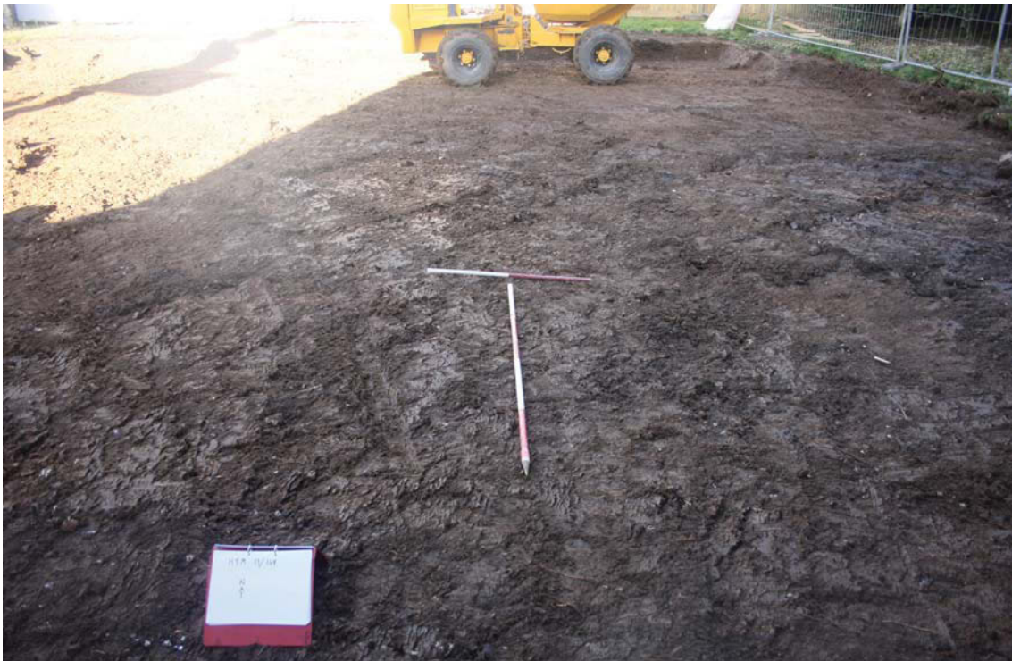
Plate 1. Overburden stripping in progress, looking north, Scales: 2m, 1m and 0.5m.
