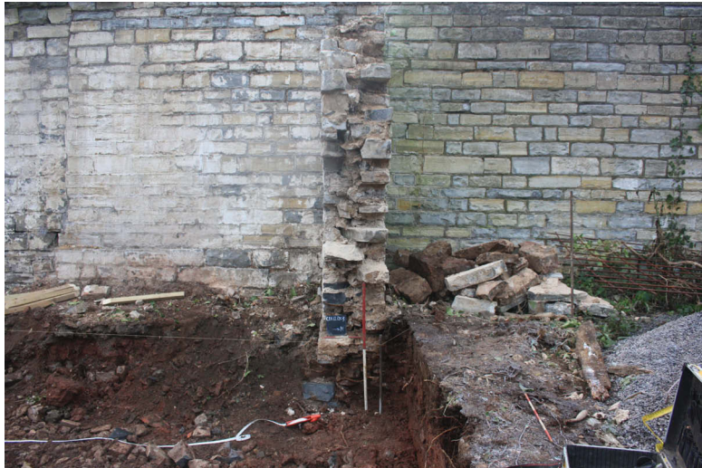
Plate 1. Wall of old outbuilding, looking west, Scale: 1m.
