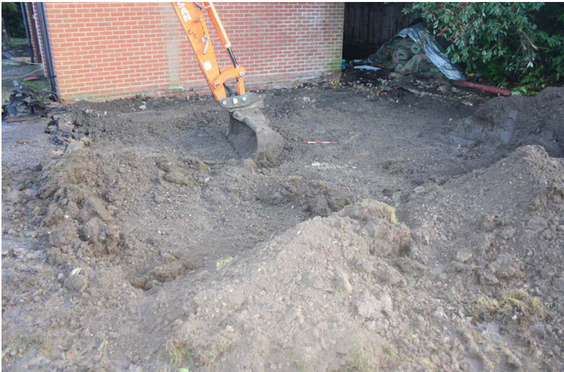
Plate 2. Strip for raft foundation at garage extension, looking north, Scale: 0.5m.
