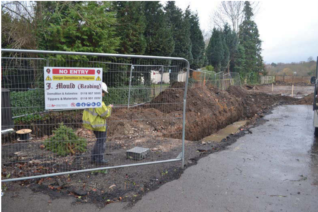
Plate 1. General view of the site, looking west.
