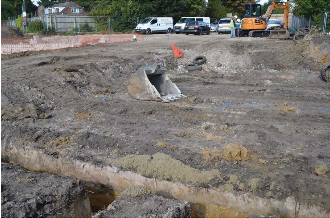
Plate 1. Block B, looking Northwest.
