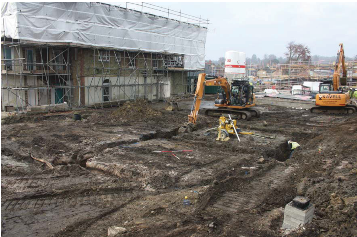
Plate 2. Block F, looking Southwest, Scales: 2m and 1m.
